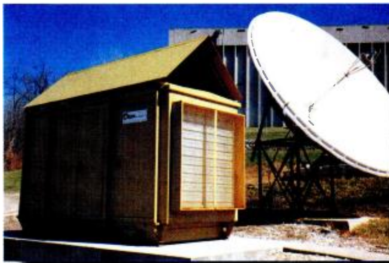
Standby generators can be reasonably self-contained, but require a stable mounting surface and considerable airflow.
